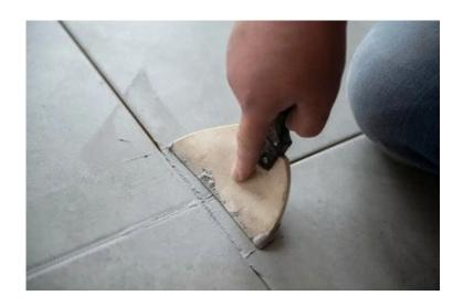
Polymer based, Un-sanded cement grout for interior & exterior, floor & wall joints of width 1mm – 3 mm
